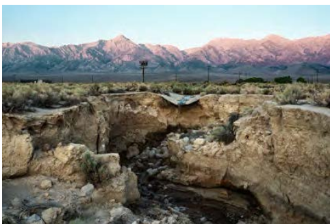
12. Symmes Creek Subsidence, Owens Valley, CA
