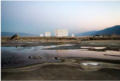
5. Water Pump for Sheet Flood Irrigation Pond, Owens Lake, CA 17.5 x 24 Inch Archival Pigment Print, 2013
