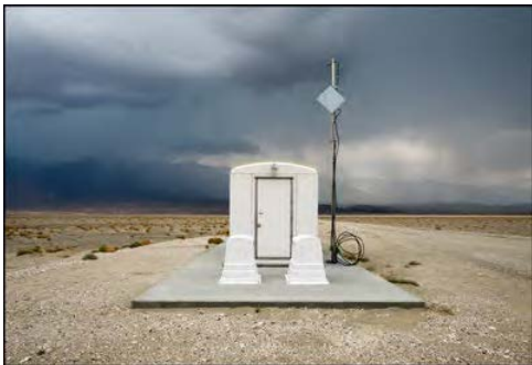
11. Small LADWP Water Pumping Station, Owens Lake, CA
