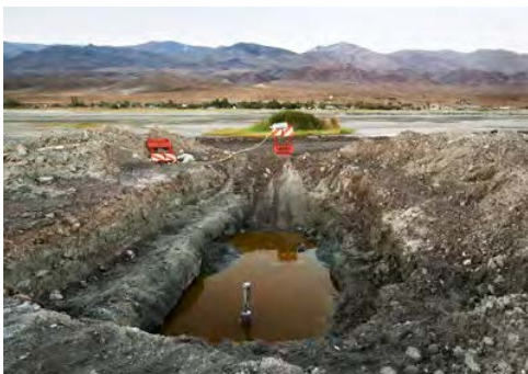
4. LADWP Irrigation Construction, Owens Lake, CA
